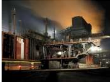
coke oven battery at night
