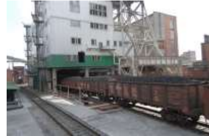
coke charging processing tower
